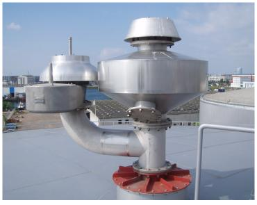
Standard Tank Vent Odour Filter in a selfcontained version, with a breater valve (pressure/vacuum) regulation, for smaller tanks.
